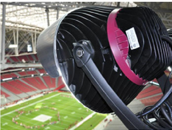
*Figure 3. Large Die Cast Heat Sinks for High Power LED Stadium Lights [3]*
